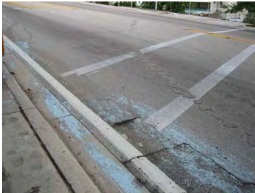
Flagler Street Bridge at SW 3 rd Court
