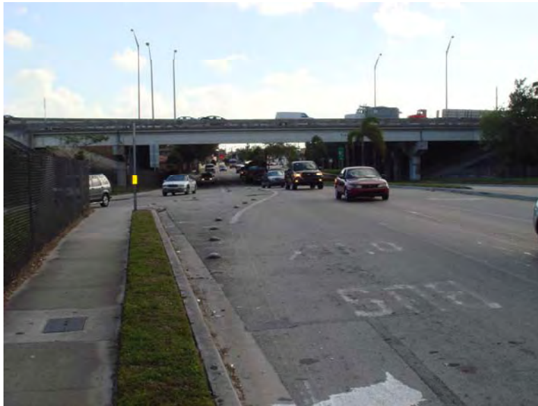
NW 17 th Avenue Northbound Lanes Narrow from Three Lanes to One Through Lane at South River Drive
