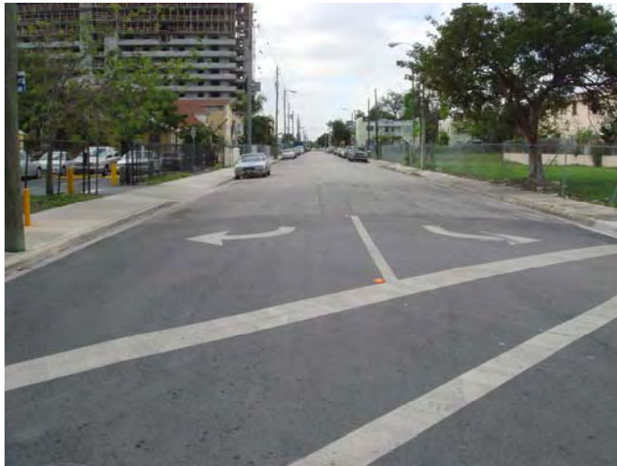
NW 1 st Street at South River Drive looking west
