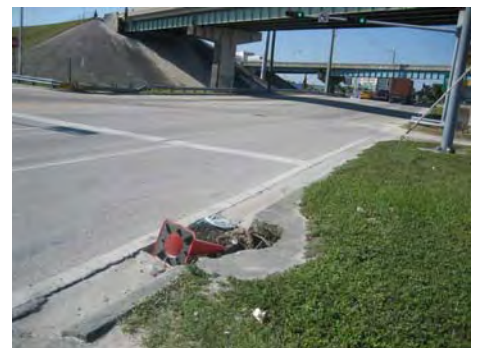
South River Drive at SR 112 Interchange
