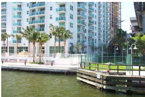
Fence on riverwalk section between Brickell on the River and 5 th Street Metromover station
