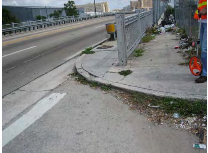
Sidewalk on South End of NW 12 th Avenue Bridge
