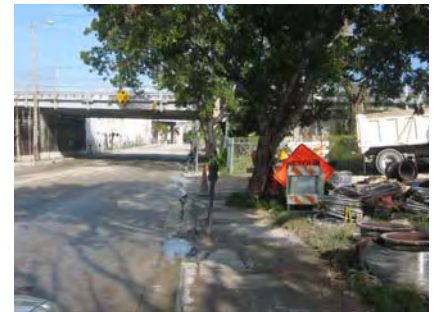
East side of North River Drive and SW 1 st Street Bridge
