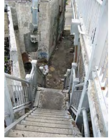
Staircase at SW 1 st Street Bridge
