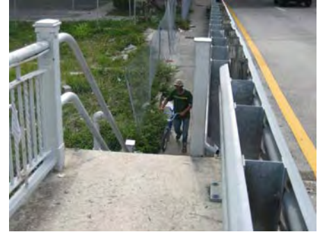
SW 1 st Street Bridge
